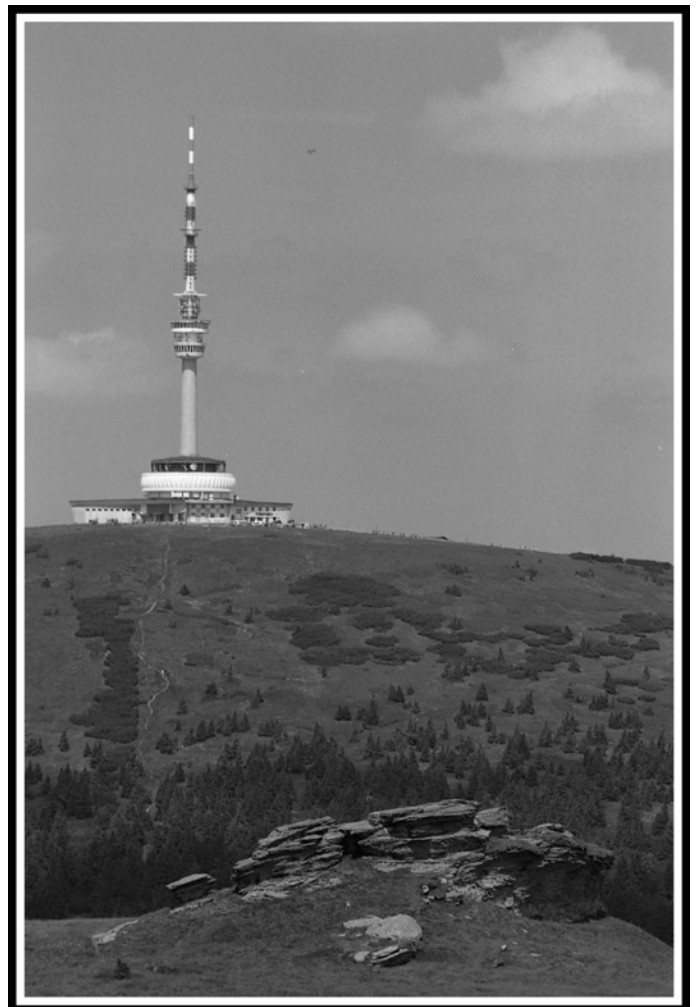
Fig. 3: The TV tower on top of the highest point in Jeseníky (Czech Republic) - Praděd (elevation 1492 m).
